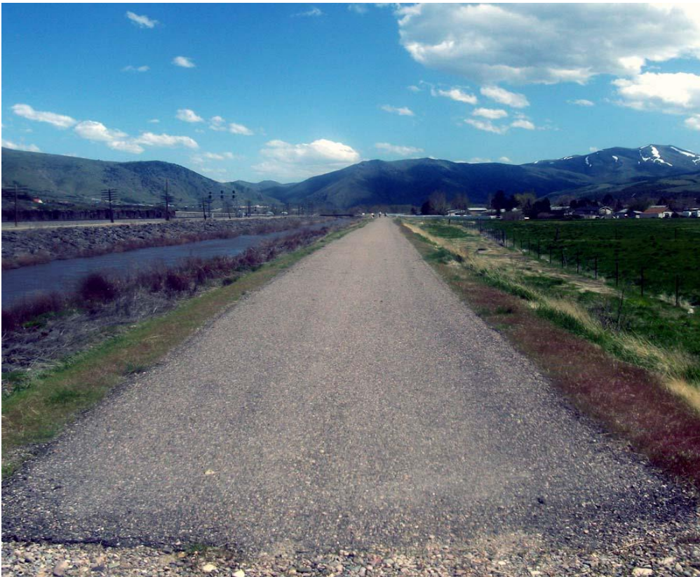
RCH6 Paved Levee Top Trail Looking South Towards Edson Fichter Nature Area
